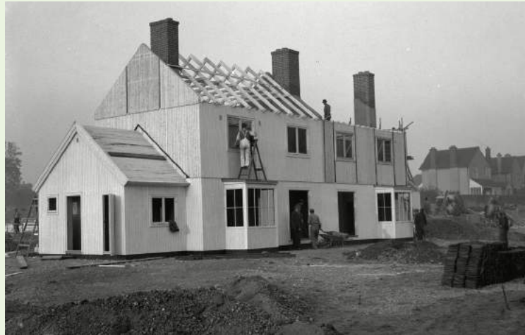
Builders, supervised by Swedish foremen, work to complete the first of six Swedish-made prefabricated timber houses, at Abbots Langley, Hertfordshire, 1945
