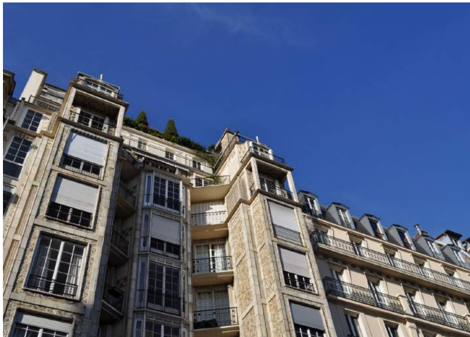
Auguste Perret, 25 Rue de Franklin, Paris, 1903. Instead of being concealed, the concrete structure (columns, beams, wall panels and floor slabs) is clearly visible on the exterior
