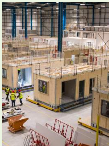
L&G Modular Homes factory in Leeds
