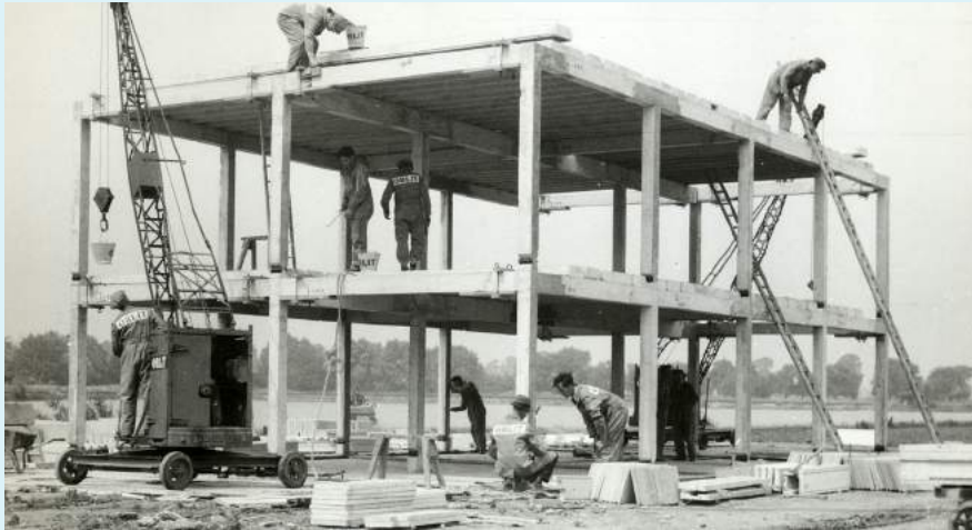
Workmen constructing the precast concrete frame of an Orlit prefabricated house, circa 1945. Seventeen thousand were built from the 1940s to 1950s. Designated defective!
