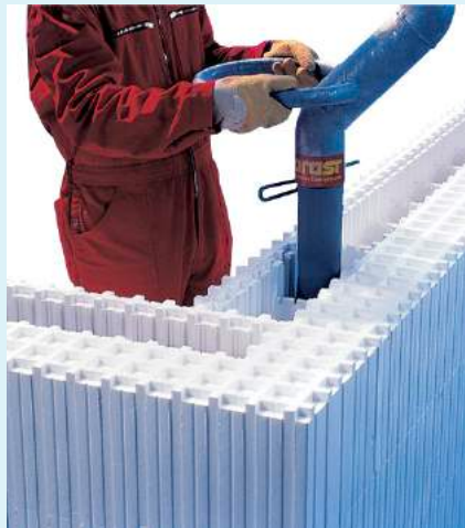
Hollow blocks of insulating material are stacked to create the mould for structural concrete walls
