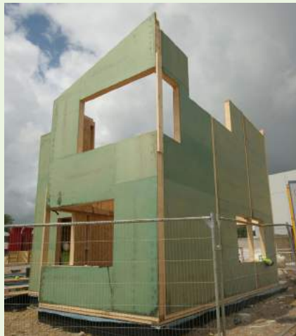
Oxley Woods panellised timber frame: complete wall panels and floor cassettes
