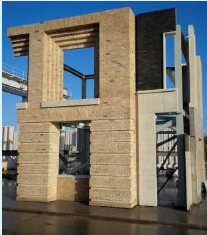
Garden Halls, Kings Cross, London, 2017, by TP Bennett/Maccreanor Lavington providing 1,200 student rooms and constructed from around 1,100 precast panels incorporating 4 brick types
