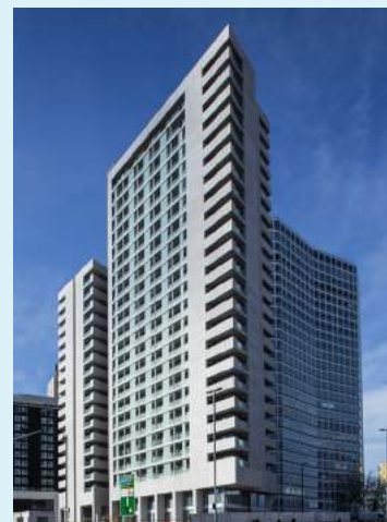
Arena Central, Birmingham, 2019 using up-to-date precast construction
