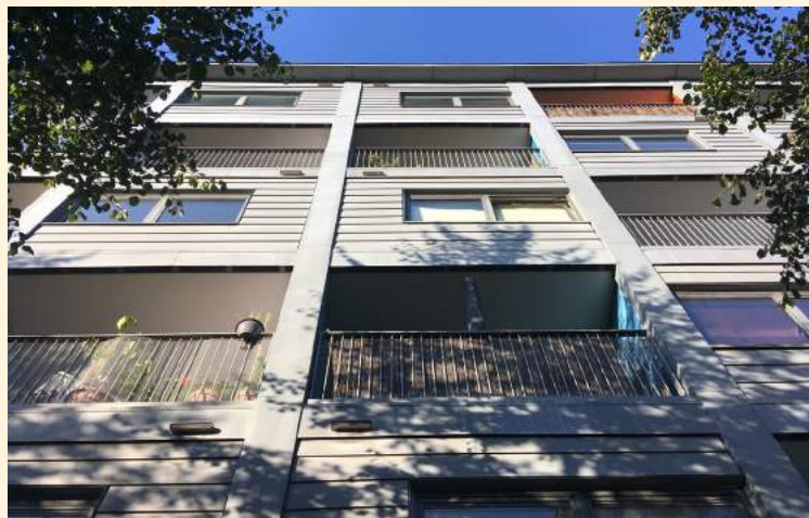
Raines Court, London, 2003 zinc façade
