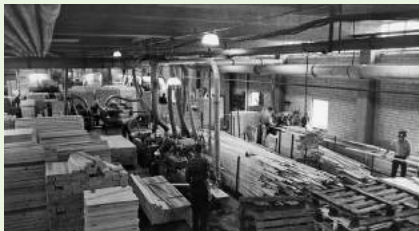
AB Elementhus factory: industrialised construction
